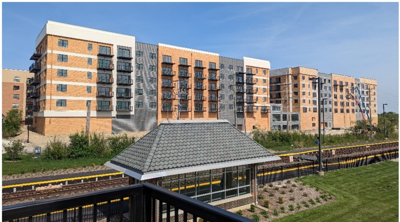
Illustration 2: D1 and D2 under construction
