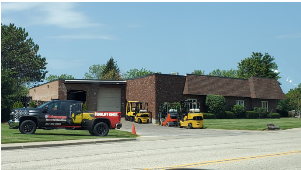
Figure 5: Image provided by Code Enforcement
