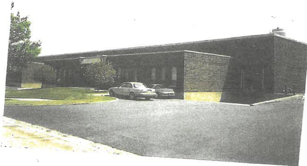
View of Front of Site From Northwest
