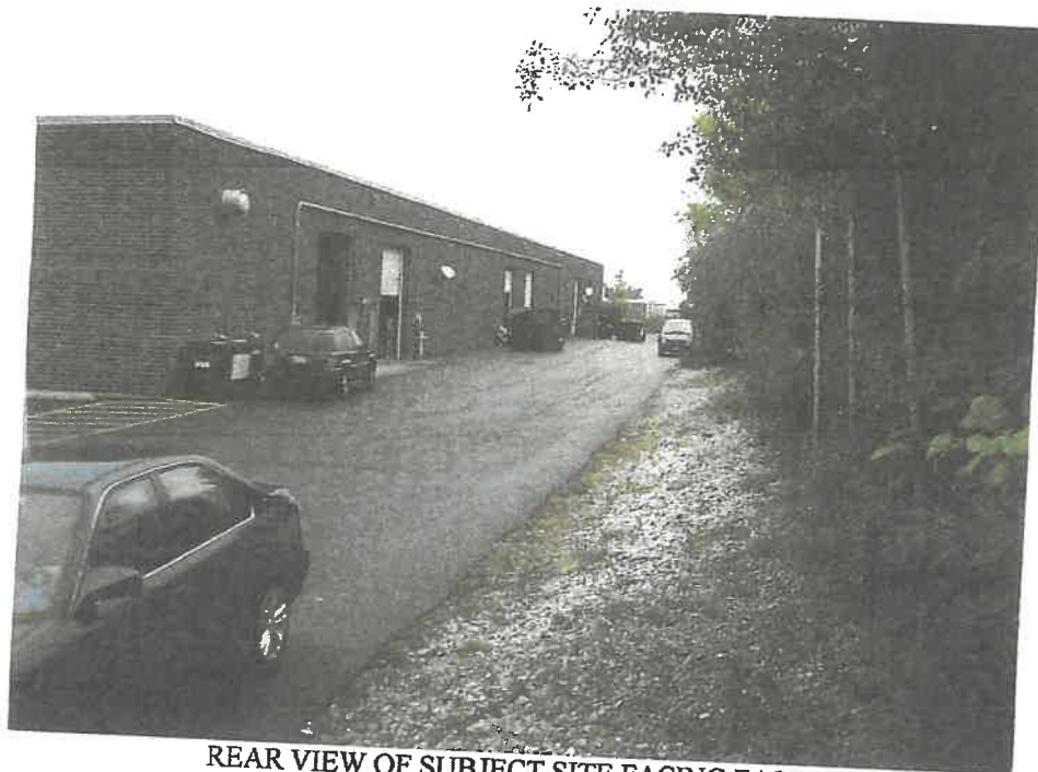
REAR VIEW OF SUB JECT SITE FACING WEST
