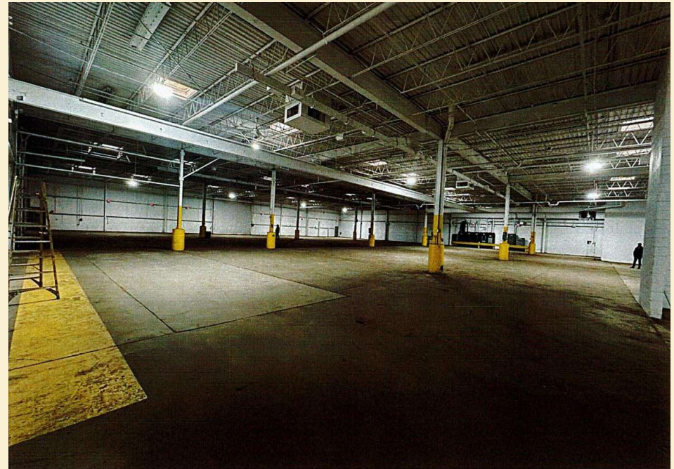
Existing Interior Conditions
