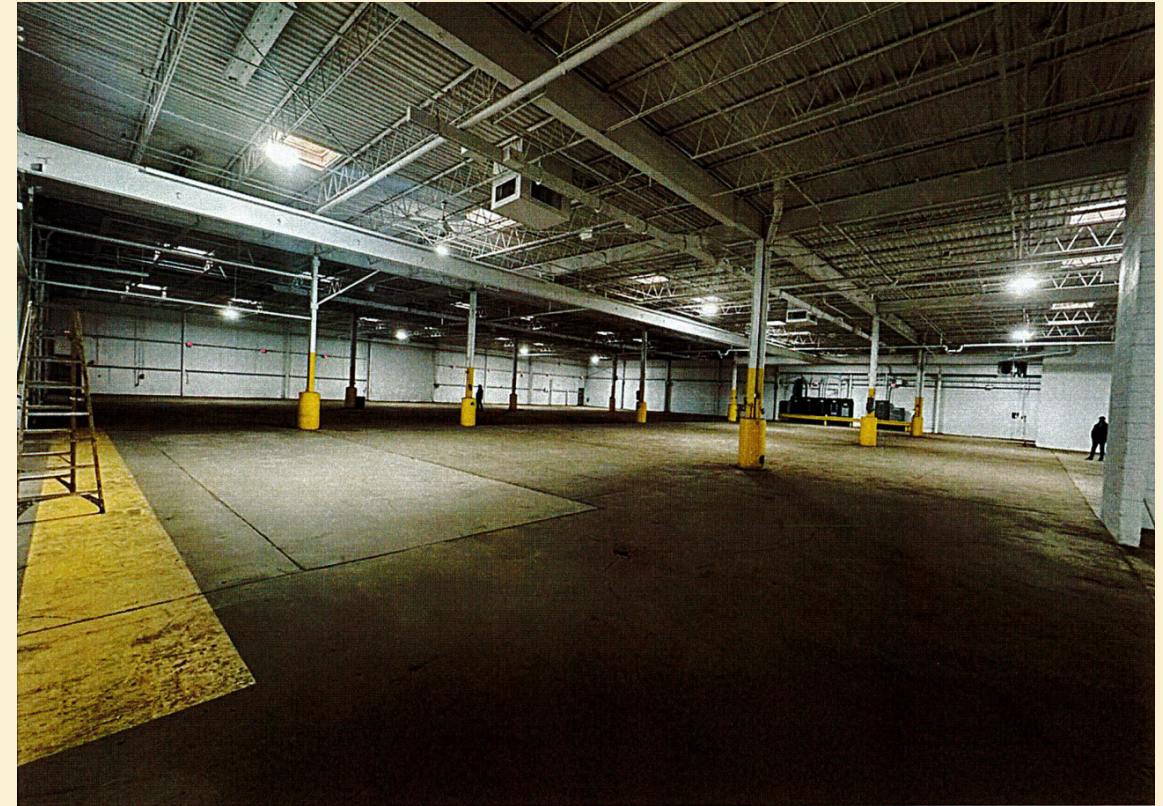
Existing Interior Conditions
