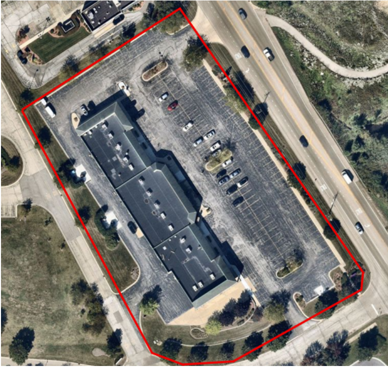
Figure 4: Aerial of the Subject Property
