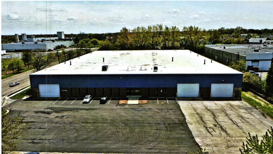
Current Parking Lot
