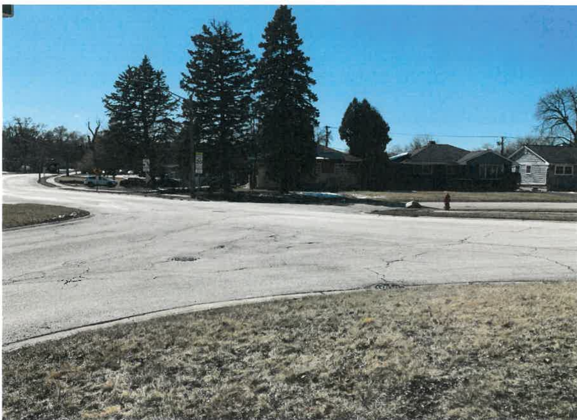
Northeast corner of the intersection
