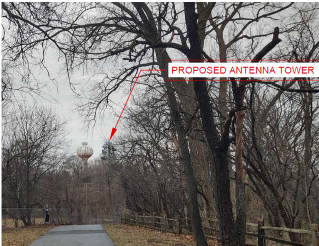
A view from the northwest looking southeast within Mundelein Seminary.
